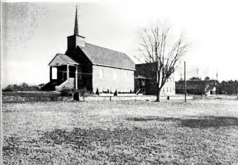
Center Grove Baptist Church Friday, October 29, 1993 9:00 A.M.
